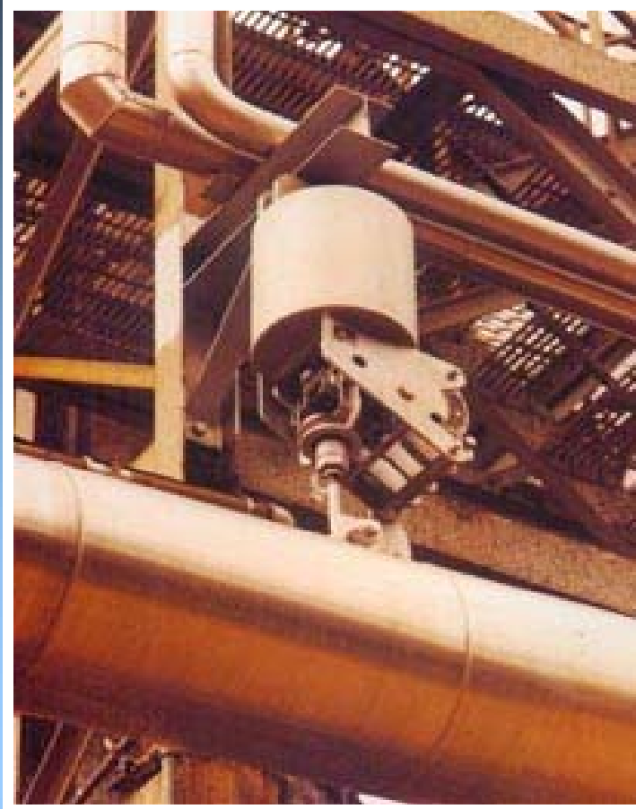
Typical Constant Pipe Support
